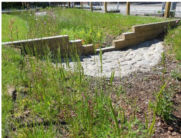
Swales - West Gorton, Manchester, gets a new park that drinks water - GrowGreen (growgreenproject.eu)
